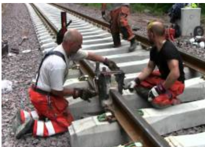
36. Railroad thermite welding
